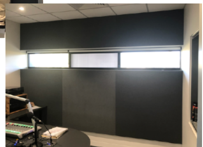
To minimise damage to the plaster, the 5 ply wood backing boards were cut to fit the walls and screwed on. The acoustic panelling was glued onto them. Below: Studio 1 finished.
